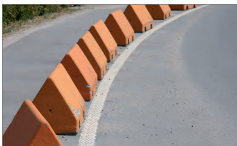
Concrete guidance elements for temporary protection of sidewalks
