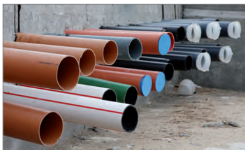
Empty conduits of a planned line route within a bridge abutment
